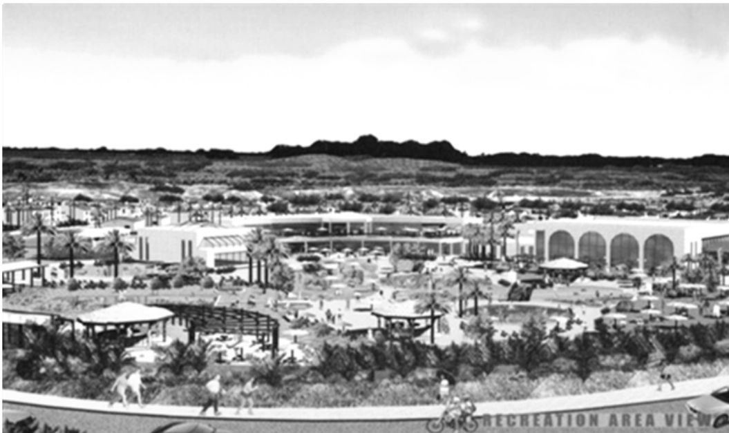
Fig. 6. The recreational area is located in the center of the project; the designer was aware of this point and located all the facilities as a cluster in the middle of the project
